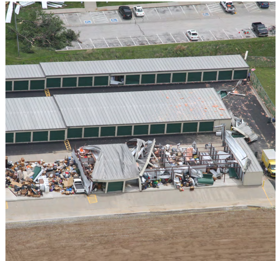
A June tornado caused damage to storage units in La Platte.
